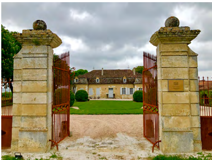
The historic Château de Vacquié in Haut-Armagnac.
