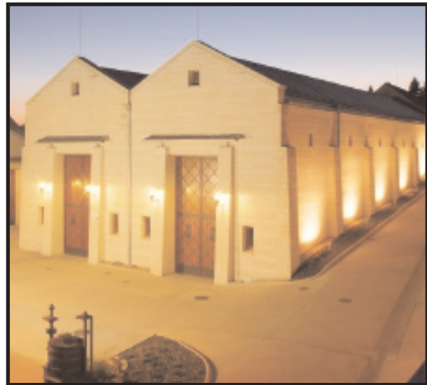
The winery buildings of The Royal Tokaji Company.
