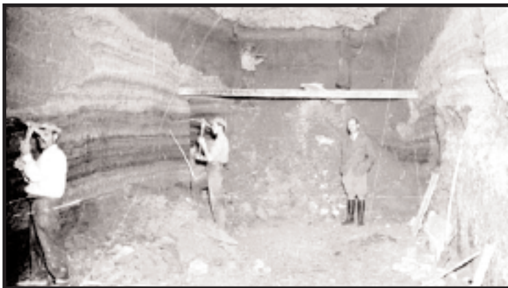
Workers digging cellars into a chalk cliff, Torre in Pietra.
