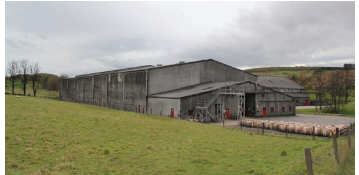
The Glendronach warehouse, Scotland.
